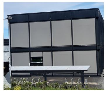
Automatic solar shading also screens view into the hub. © Lillin Catherine Knudtzon
